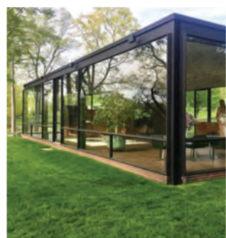
#theglasshouse honored to be on the advisory board of this legendary 1949 #philipjohnson beauty
